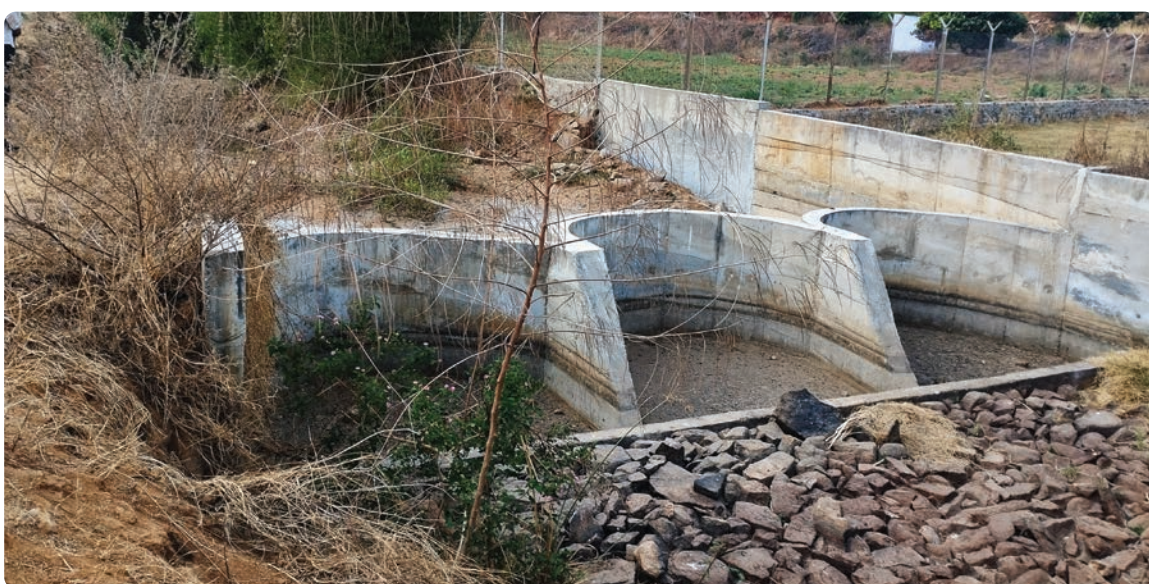
Water harvesting structures built under Sanjeevini
