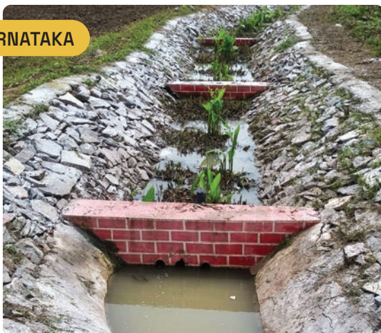
Well maintained Inline Treatment System in Bedavatti Village, Shirur GP, Yelburga Block in Koppal District, Karnataka
