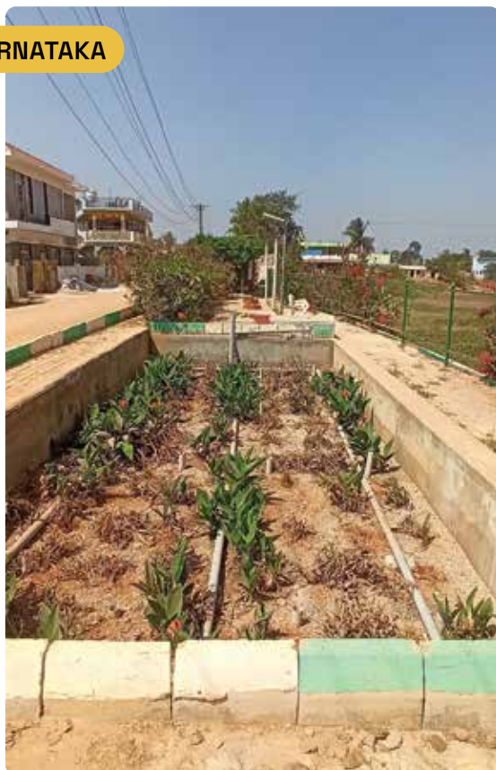
Constructed Wetlands with DEWATS in Muthur Village, Sidlaghatta taluka of Chikballapur district, Karnataka
