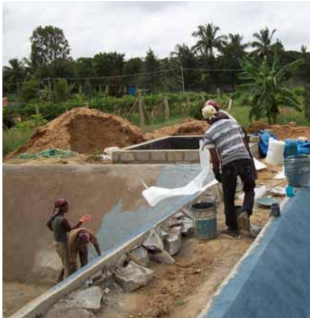
Construction of the SBT plant at ACCEPT
